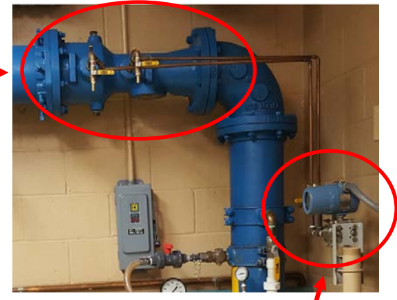
Differential Pressure (DP) cell, or transmitter
