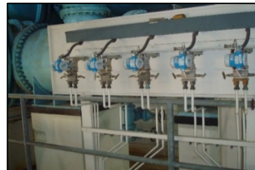
Bank of Differential Pressure Cells connected to flowmeters (Courtesy of Louisville Water Company)
