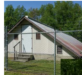
Covered water storage reservoir in a small system in Pennsylvania
