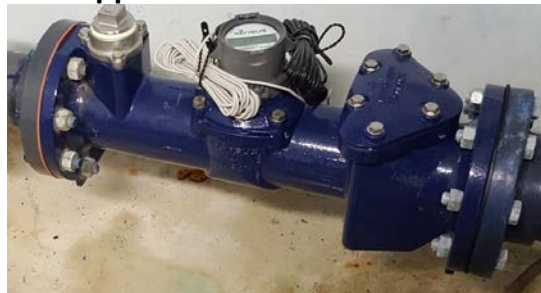
4-inch floating ball turbine meter installed in 2018
