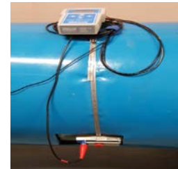
Portable strap-on ultrasonic meter to measure flow to compare with host meter
