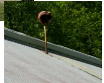
Visible floating ball indicates a full reservoir level – a lowered ball indicates a high water demand (as from a leak)
