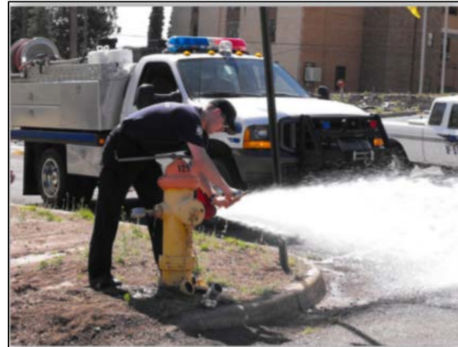
Fire hydrant flushing
