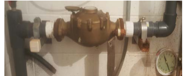
Upstream and downstream 90-degree bends cramp 2-inch turbine meter layout
