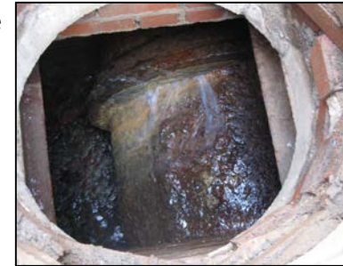
Cast Iron pipe joint leak
